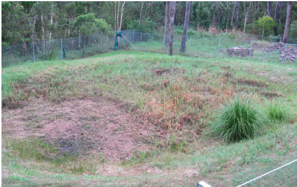
Figure 21 Existing On-site Detention System
